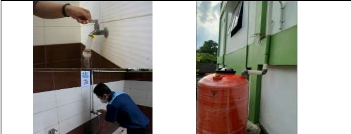
Reservoir of water used for ablution to be reused at the USU Faculty of Medicine
