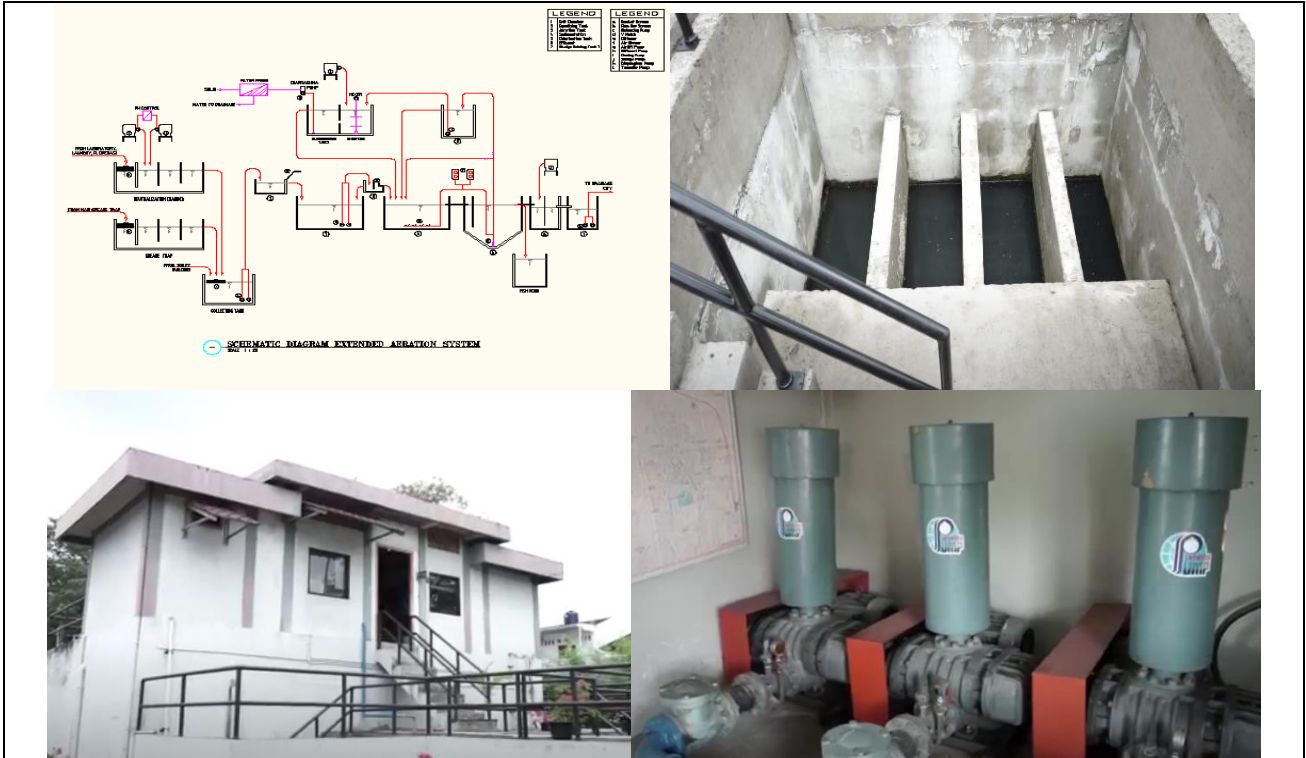
2. Waste Water Treatment Plant at USU Hospital
