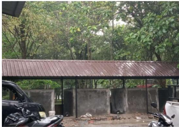
1c. Compost processing building consisting of 4 compartments to process organic waste
